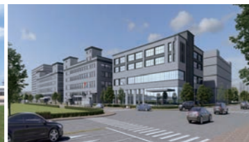
High-tech Zone factory
